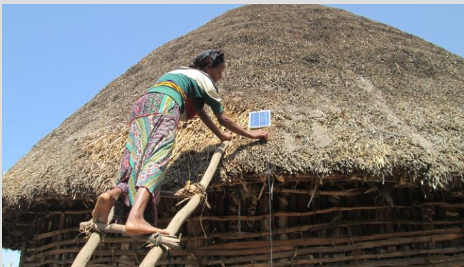
A woman installing a small solar PV system
